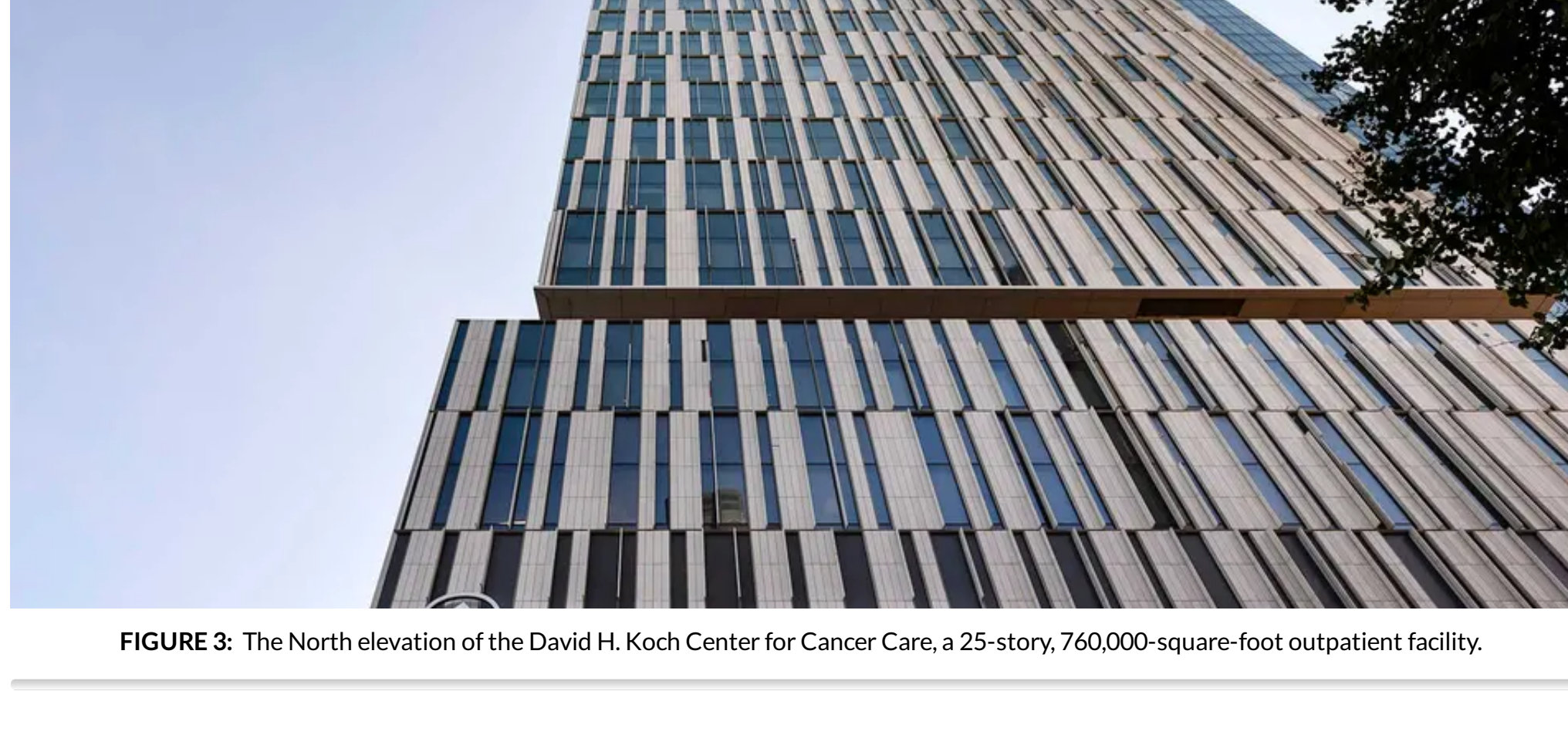
FIGURE 3: The North elevation of the David H. Koch Center for Cancer Care, a 25-story, 760,000-square-foot outpatient facility.
